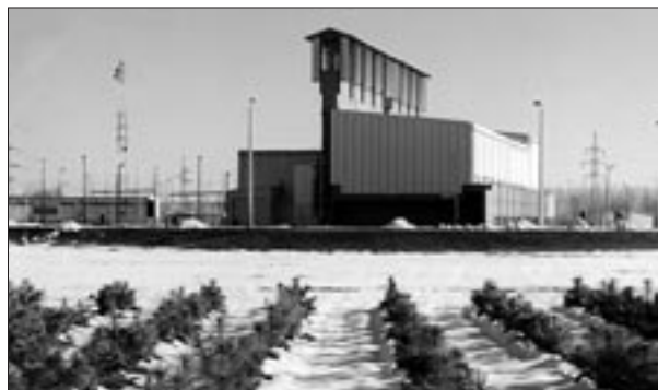
Interim Storage Facility for Spent Fuel (ISFS), Paks NPP.
