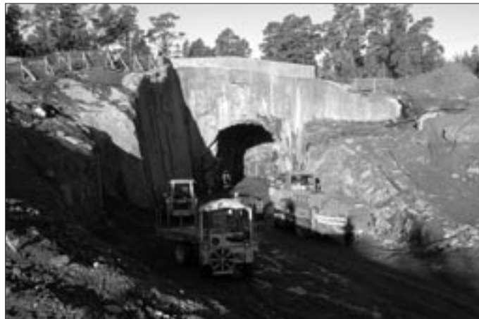
ONKALO underground repository. Posiva Oy, Finland.
