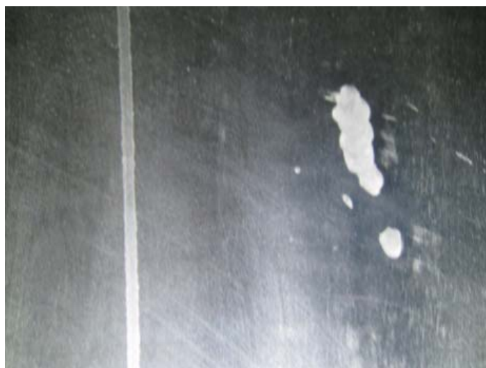
Hot leg weld root and a base material weld repair.
