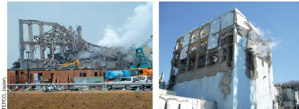
Fukushima Daiichi units' 3 and 4 damage after hydrogen explosion.
