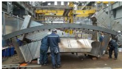
Part of BU under welding
