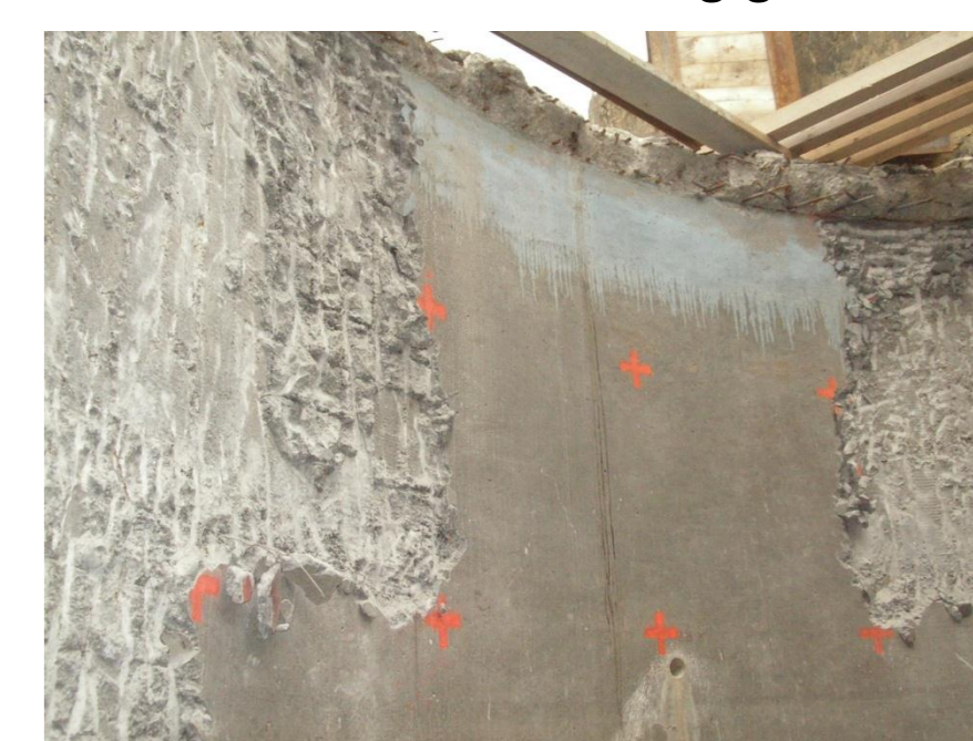
Fig. 6 Example of decontaminated and non-decontaminated internal concrete surface of tank with demarcated monitoring grid
