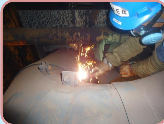
Cutting by a plasma cutting machine
