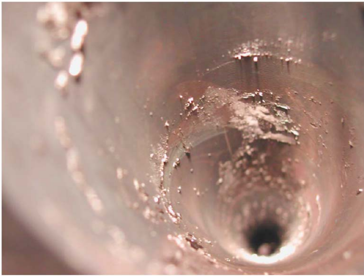
Fig. 4(a). Interior of the pipe after the first run at low oxygen concentration.
