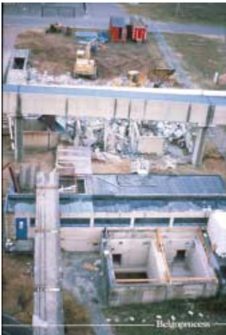
Figure 1. Demolition of buildings 6A/6B
