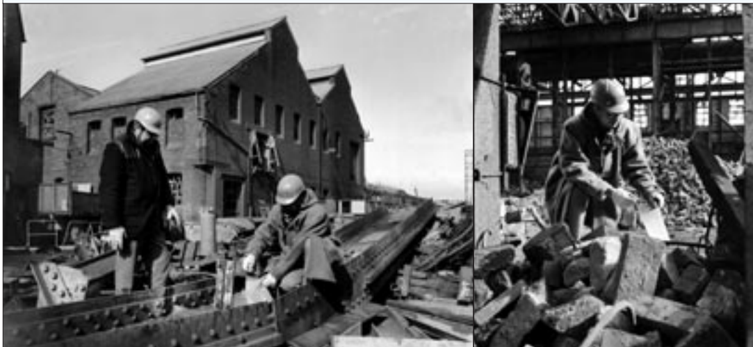
The radiation protection system has evolved over the years. The photos here show workers in the 1970s checking for release of toxic material during cutting-up operations on steelwork, and sampling firebrick from a demolished furnace at Harwell in the United Kingdom.
