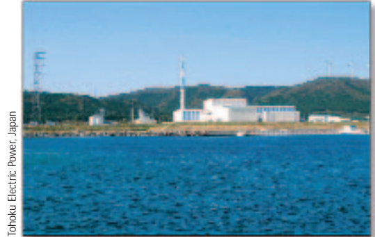
View of the Higashidori-1 nuclear power plant, Japan.
