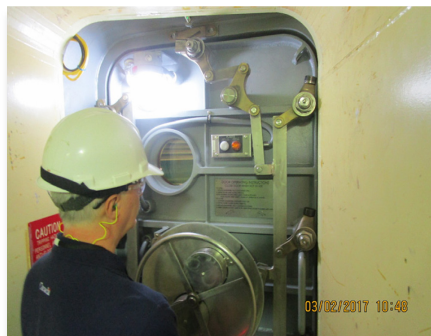
Figure 4.5: Interior of the third PAL door in the reactor building
