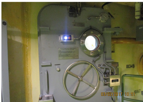
Figure 4.4: Exterior of the third PAL door in the reactor building
