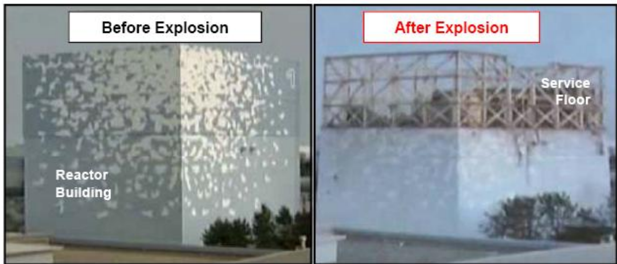
Figure I.4 Condition of the reactor building of unit 1 before and after the hydrogen explosion
